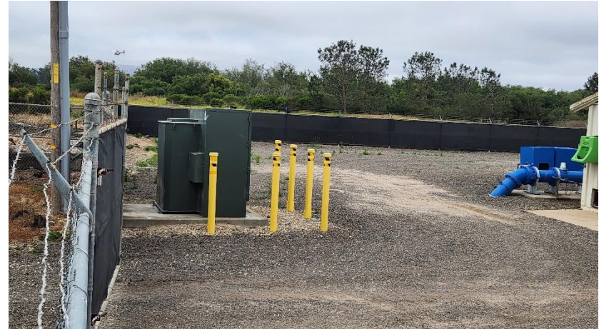
Photograph 6. Pad-mounted transformer inside fenced well enclosure in eastern portion of subject property
