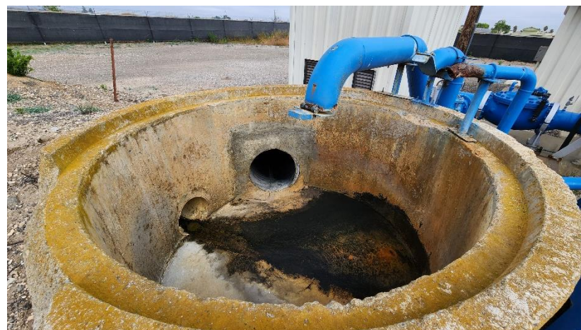
Photograph 4. Discharge basin for flushing the well, connected to stormwater system in eastern portion of subject property
