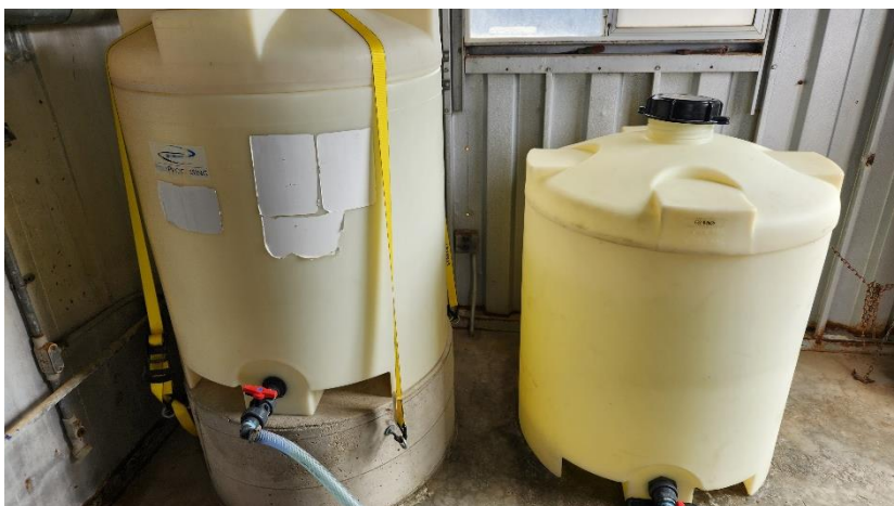
Photograph 3. 100-gallon chlorine tanks in well pump housing in eastern portion of subject property
