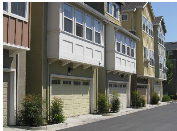
Location and design of rowhouse garage doors for tuck-under parking along alleys.
