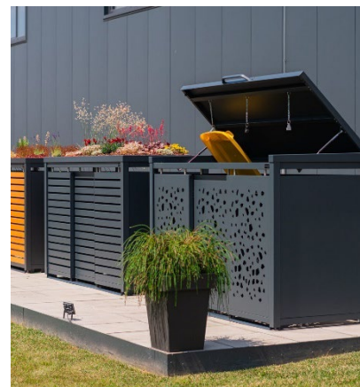
Refuse enclosure matches style and materials used on the primary buildings.
