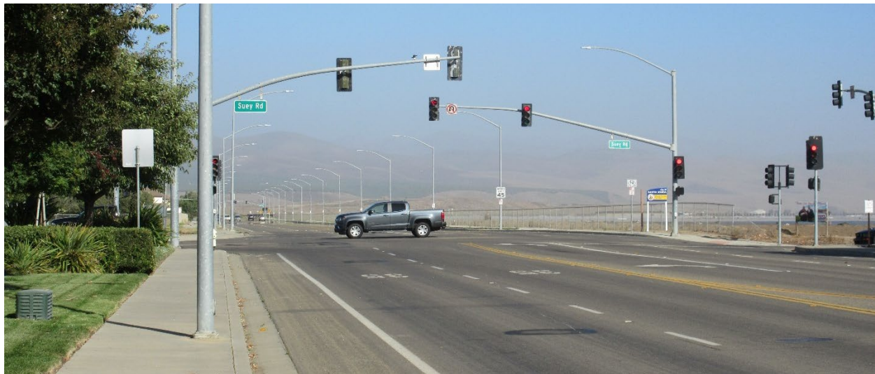
Wide roads and limited pedestrian crossings limit walkability.
