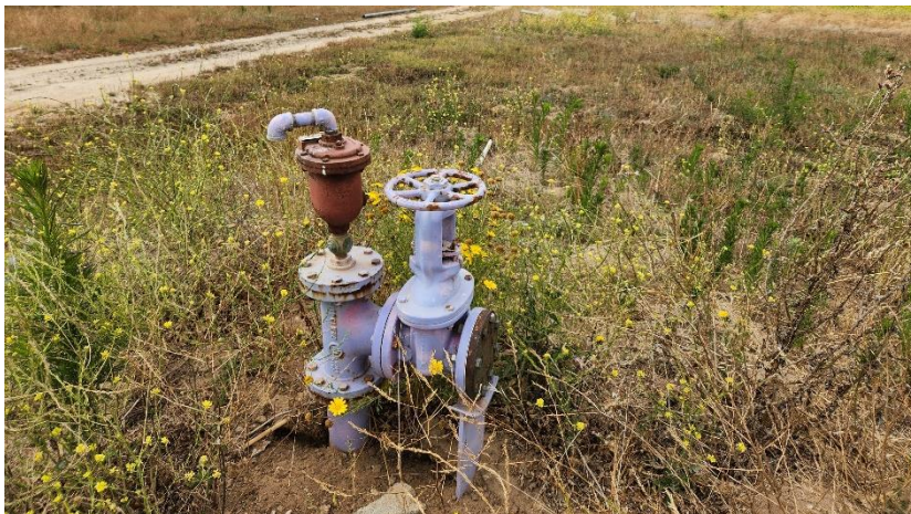
Photograph 7. Abandoned/remnant well structure in eastern portion of subject property
